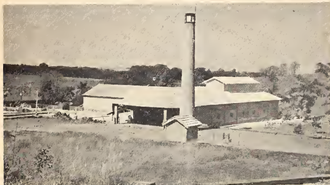
Starch plant building, on the Fazenda Santa Cruz, São Paulo. The entire plant, planned to produce ten tons of starch per day, cost about $60,000 early in 1941. Equipment, made in Brazil, was copied from European designs.
